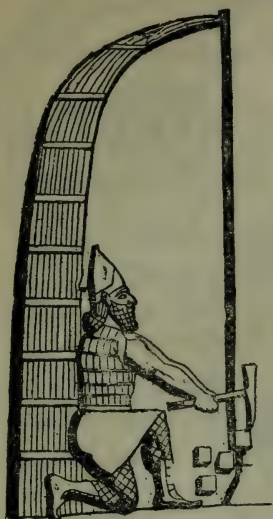
Soldier undermining a wall, sheltered by gerrhon .
